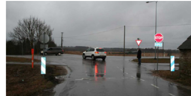
Tilgu Road's compulsory signs in front of the non-motorised road traffic crossroads (including the STOP sign) and at the highway itself (where there is a GIVE WAY sign) (CPTED course participant's photo).
