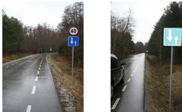
Tilgu Road's speed limit signs. The road is very narrow with no broken white lines to indicate its centre. Broken white lines (see 923b) have been laid out on both sides of the road but their purpose is not generally understood by road users. (CPTED course participant's photo).
